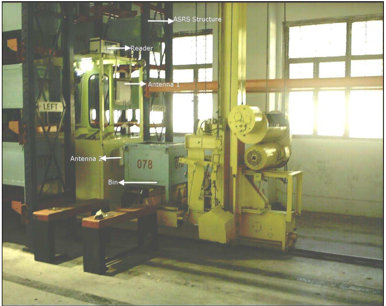
Figure 4: RFID infrastructure mounted on the ASRS
